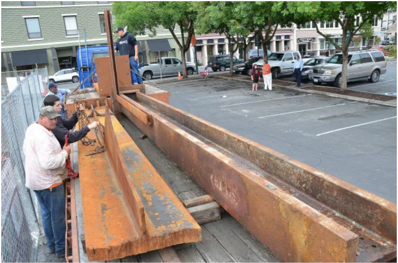
Steel beams from the World Trade Center, which were incorporated into the Napa 9/11 Memorial, arrived at the memorial site on Main Street on Tuesday afternoon, June 25, 2013, and were erected the next morning.
