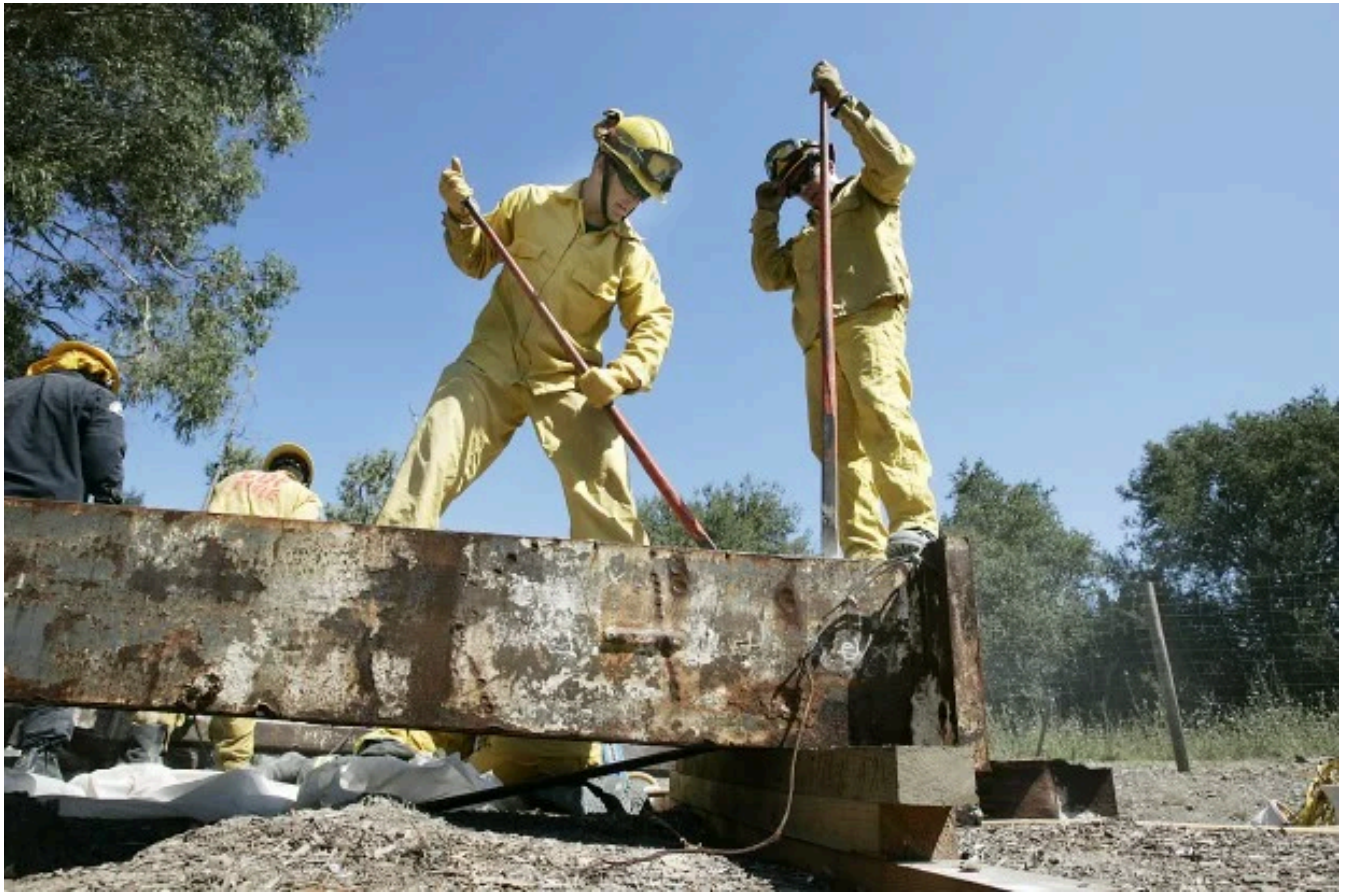
Local firefighters worked on Sept. 1, 2011, on removing debris from the steel beams to be used in the Napa 9/11 Memorial Garden, which the artist Gordon Huether created from materials from the World Trade Center.
