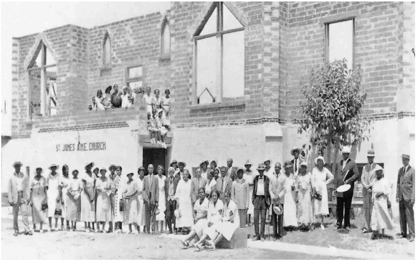
The congregation of St. James AME at its current location on Richter Street during construction. Courtesy of St. James AME
