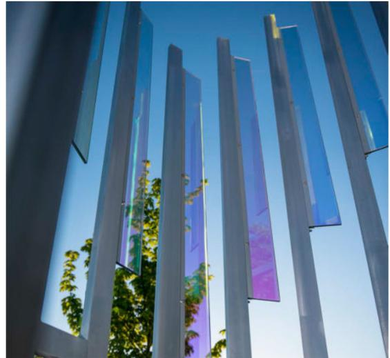
*Colored glass strips attached to the extruded aluminum lengths filter light and the surrounding environment.*
