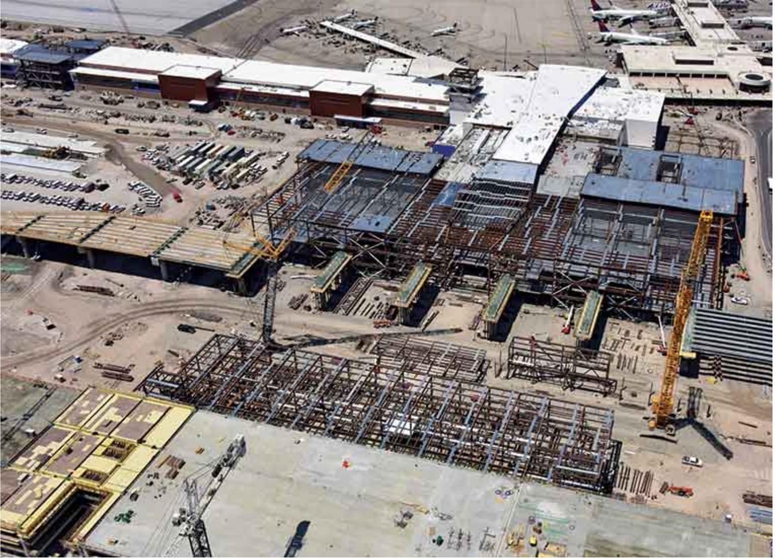
Two sky bridges will connect the parking garage to the second level of the terminal, while an elevated roadway for departures will access the third level. Six miles of baggage handling belts will move luggage from multiple check-in points.
